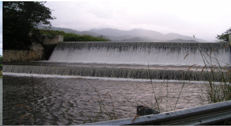
Water Dam Flood Gate Control
