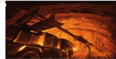
• Tunnel and base constructor
