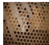
A badly scaled/fouled heat exchanger
